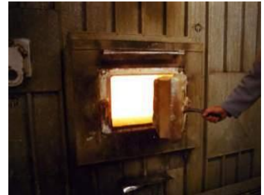
Co-generation plant at Mainz coffee factory, Germany, where spent coffee grounds are used as fuel
